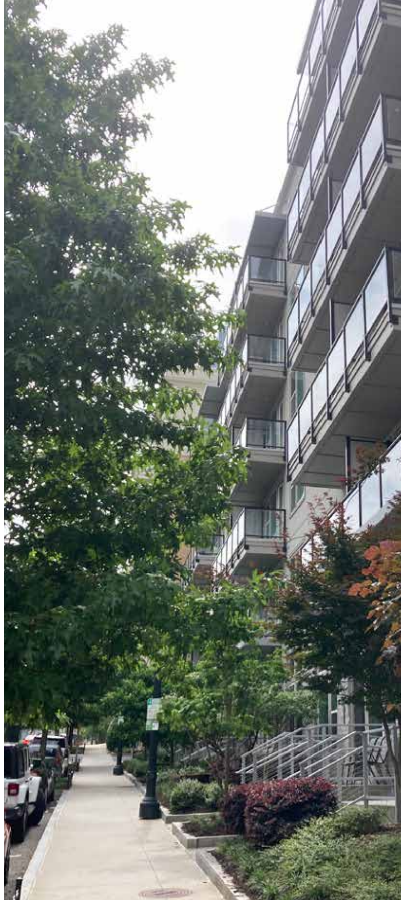
New development in many parts of the city requires a Special Administrative Permit (SAP), including these new apartments in Downtown
